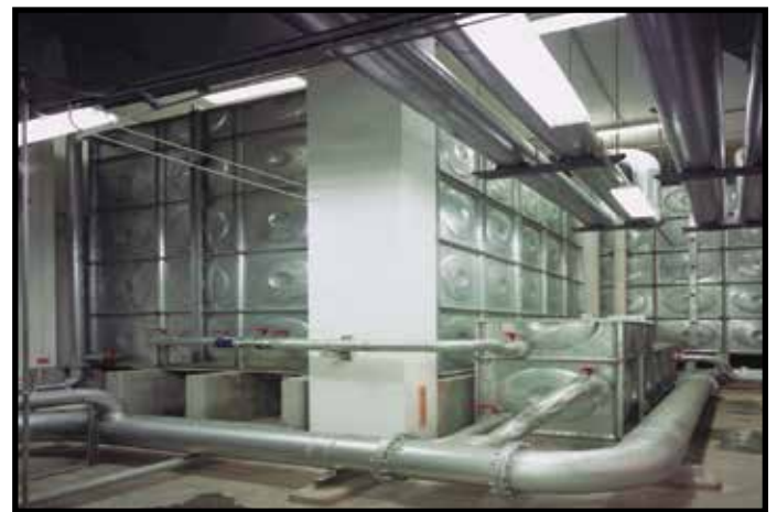
Half Panels and special cut out to accommodate obstructions.
