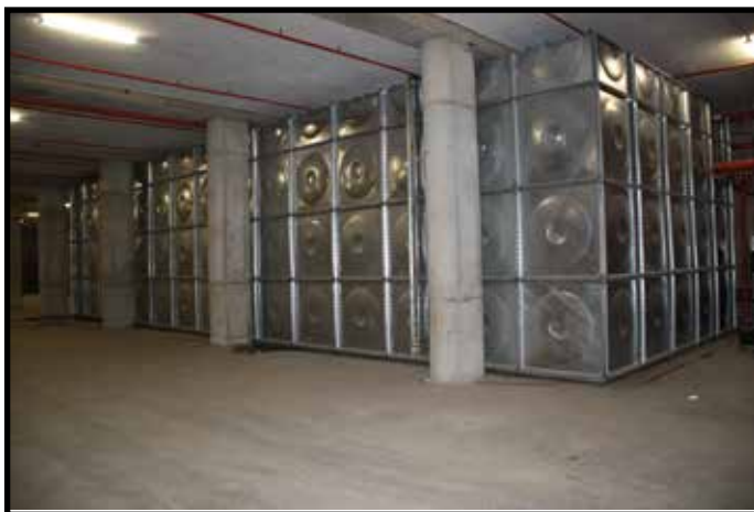
Internally bolted floor to accommodate height restriction.
