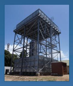
Elevated tanks are manufactured in accordance to SANS 10162-1 & 2, ensuring the highest standards. The height of elevation is dependent on the client request. Walkways and landings are supplied with elevated tanks that are 12m and higher. Customised stands can also be supplied as per the site conditions or requirements. They are commonly founded on reinforced concrete bases.
